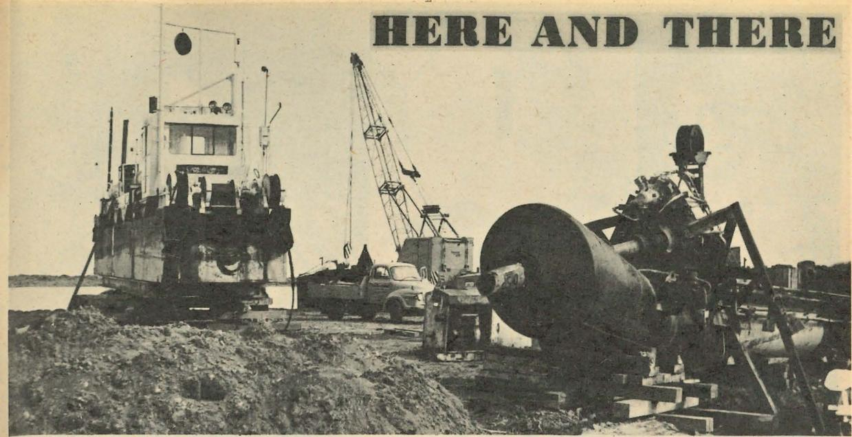
Above: All set to go. Fletcher Construction's suction dredge all ready to be put into the water to cut a ditch across the bottom of the Wanganui River in which to lay the Kapuni gas pipeline. There was a bit of delay getting started here as the "sucker-upper" nozzle wasn't long enough to do our river.
